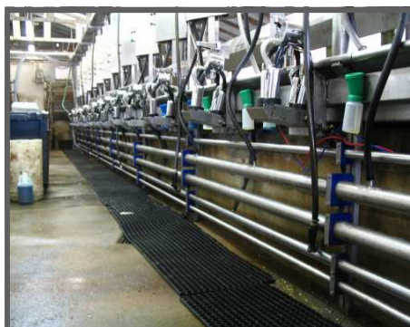
3" Lo-Lines, (2) Receiver Groups, 2" CIP & miscellaneous other Lines
