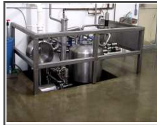
With the CIP-Receiver Combination group installed in the Milk House, there's nothing left to install in the BreezeWay
